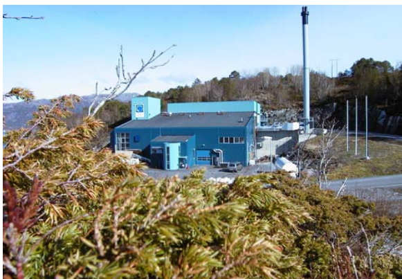
Photo: A Gasification plant, Norway
