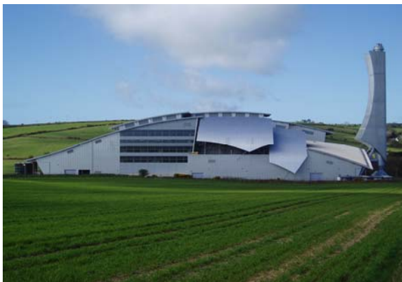
Photo: Isle of Man EfW facility
