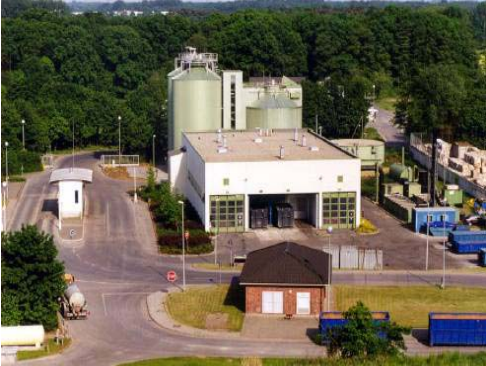
Photo: Anaerobic Digester
