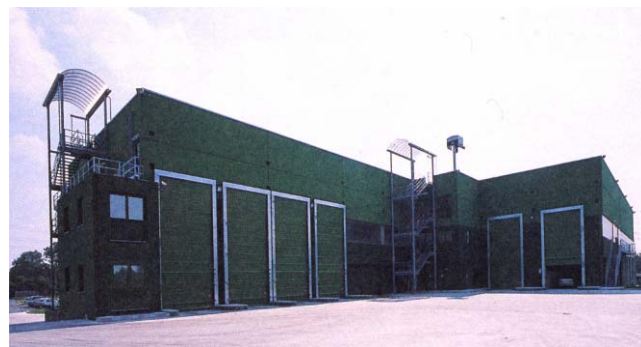
Photo: Refuse Derived Fuel MBT plant in Italy
