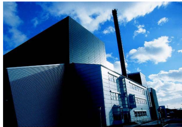
Photo: A Danish EFW Facility
